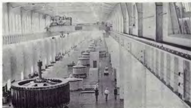
Above: Inside one of the generating stations looking down on the turbine tops.
