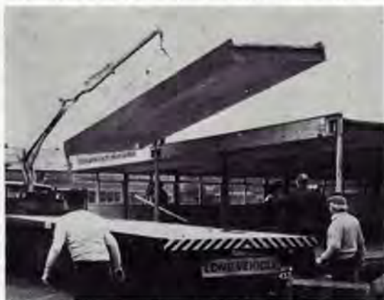
District Engineer, Mr. A. W. Hawley supervises the removal of a roof section on to a waiting lorry.
