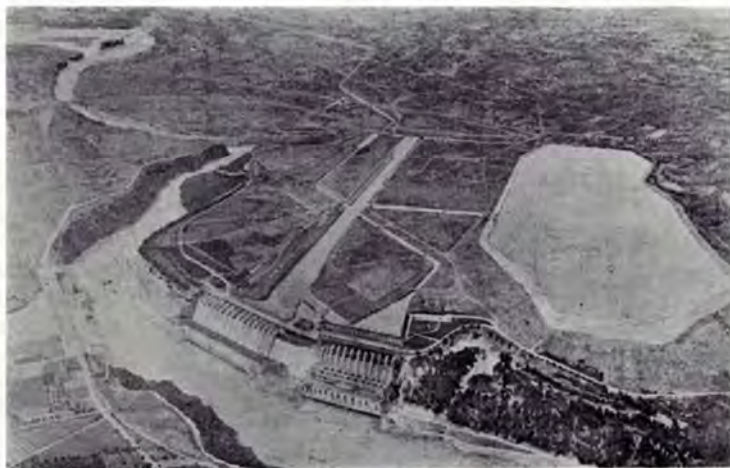
Below: An aerial view of the Sir Adam Beck dual generating stations.
