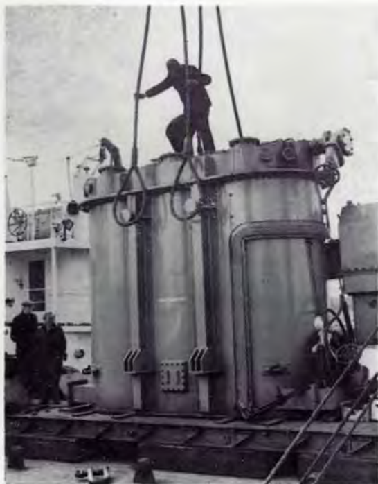
Off-loading at Holyhead—preparing to lift the huge transformer tank from the ship.
